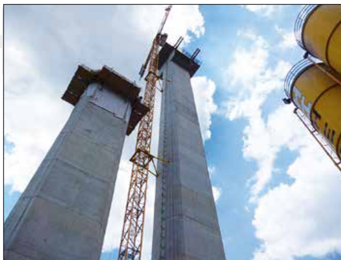
Figure 9. Concrete pump S3 right, Studenčica Bridge
