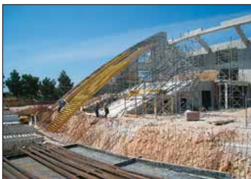
Figure 8. Placing of formwork and scaffold
