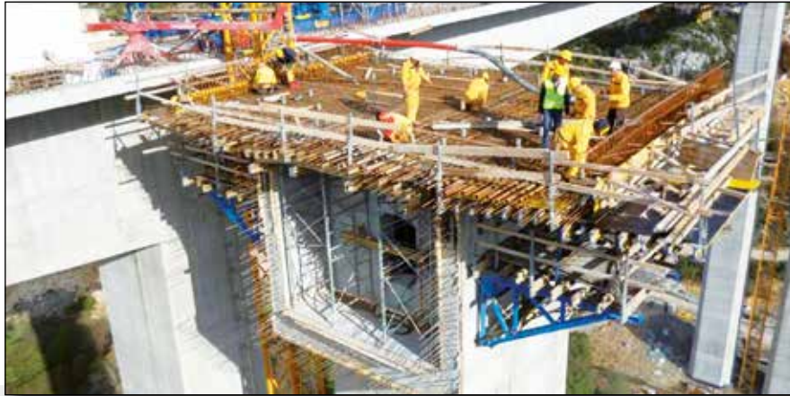
Figure 6. Construction stage, execution of base segment of span structure
