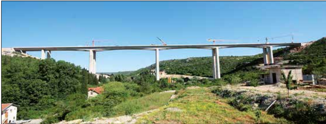
Figure 1. Studenčica Bridge, a reinforced-concrete structure, motorway, corridor 5c
