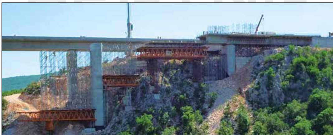
Figure 4. Construction stage, construction of span structure of Trebižat bridge on scaffolding
