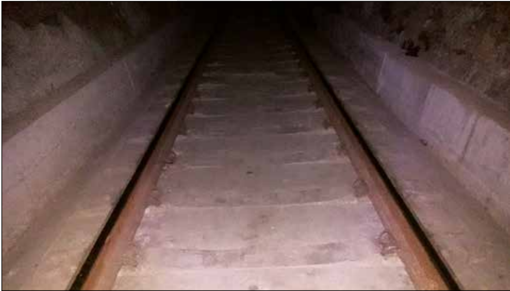
Figure 12. - RC slab in Ivan tunnel
