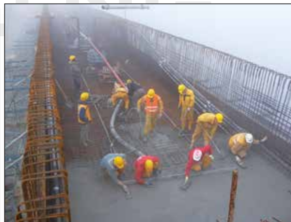
Figure 13 and 14. Concreting span structure constructed by balanced free cantilevering and on scaffolding
