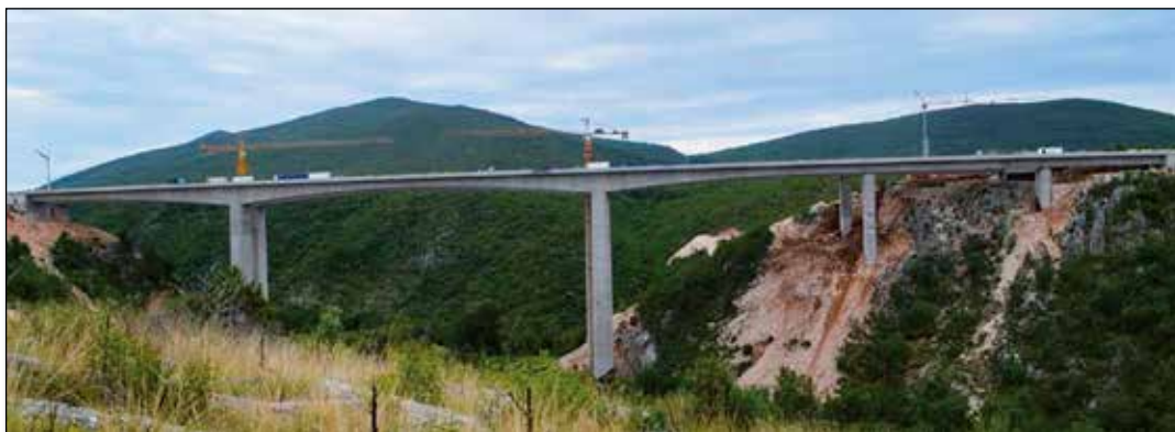
Figure 3. Trebižat Bridge, a reinforced-concrete structure, motorway, corridor 5C
