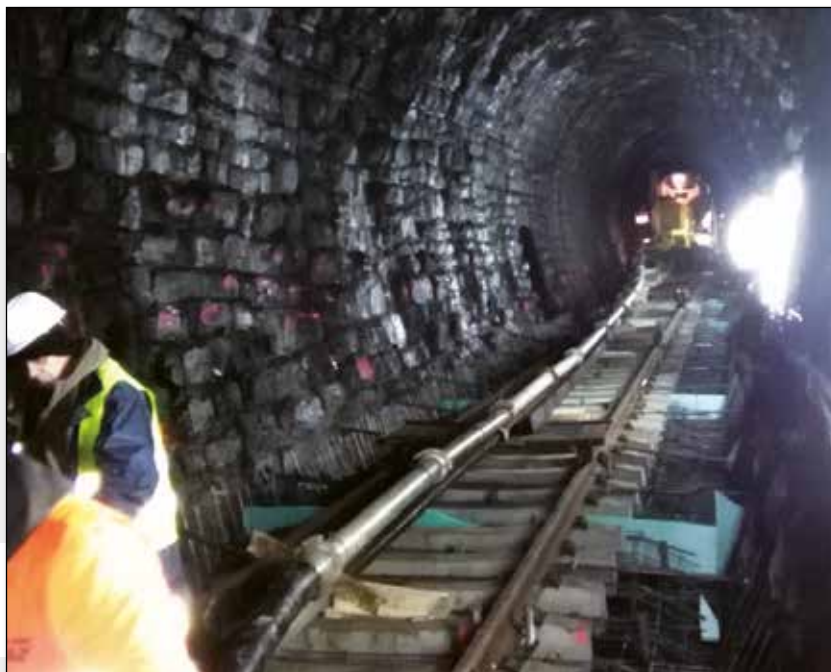
Figure 7. - Concrete transported to the location of placing
