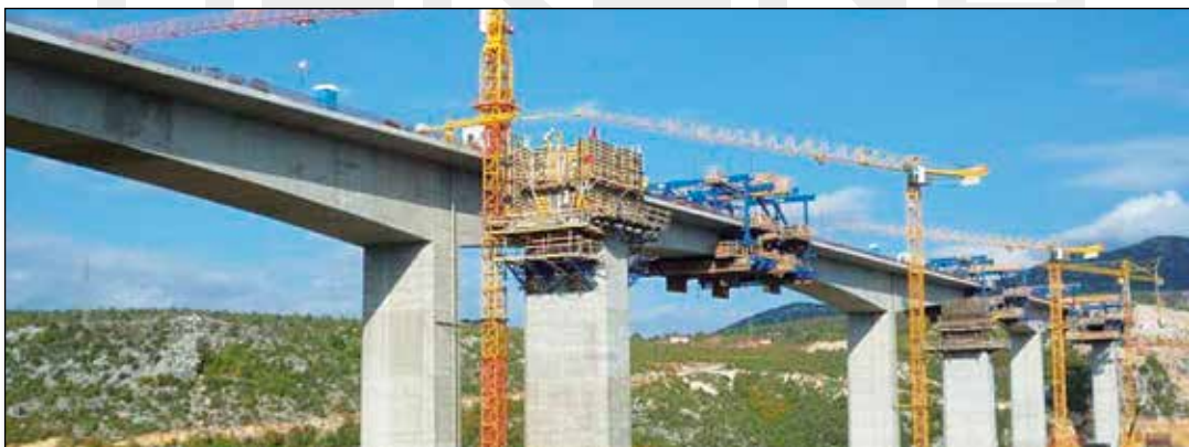
Picture 2. Studenčica Bridge, construction stage
