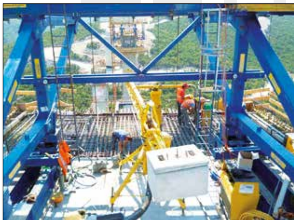
Figure 13 and 14. Concreting span structure constructed by balanced free cantilevering and on scaffolding
