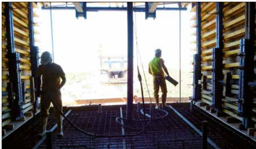
Figure 12. Concreting of segment lower slab in formwork of balanced free cantilevering
