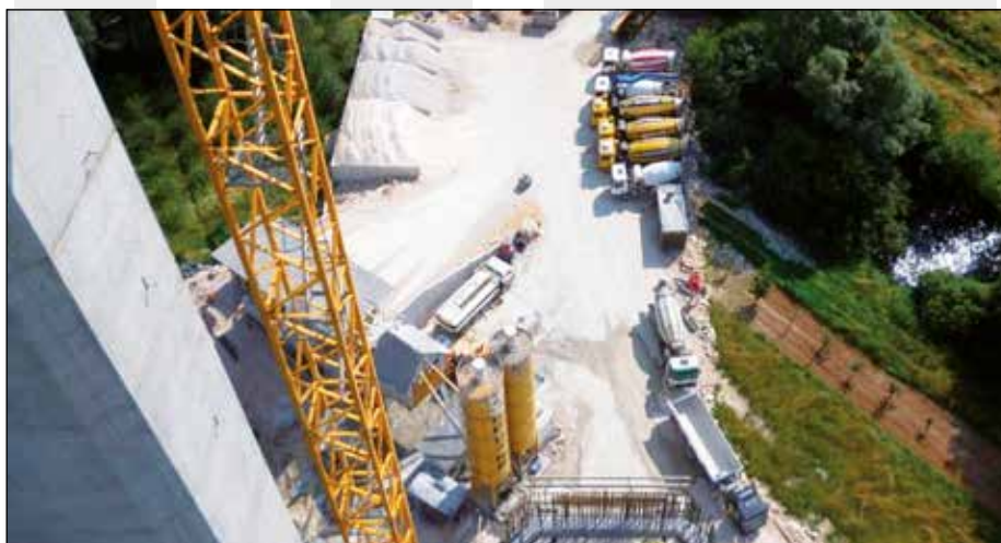
Figure 5. Concrete batching plant on a construction site of Studenčica Bridge
