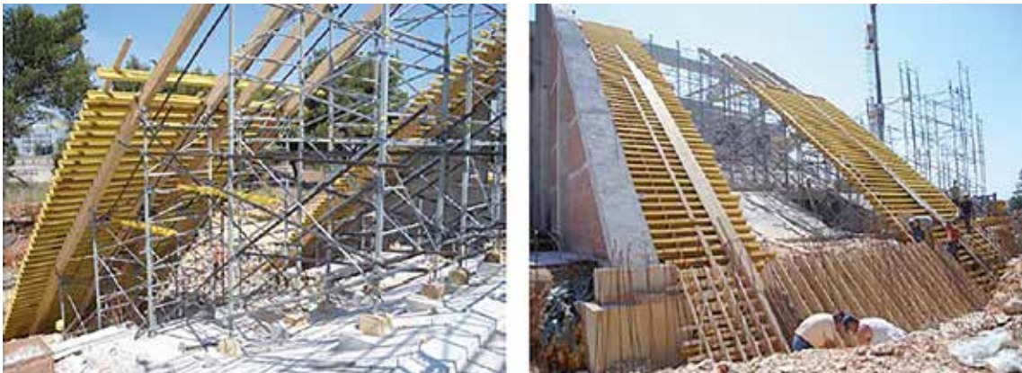
Figure 9. Placing of formwork and scaffold
