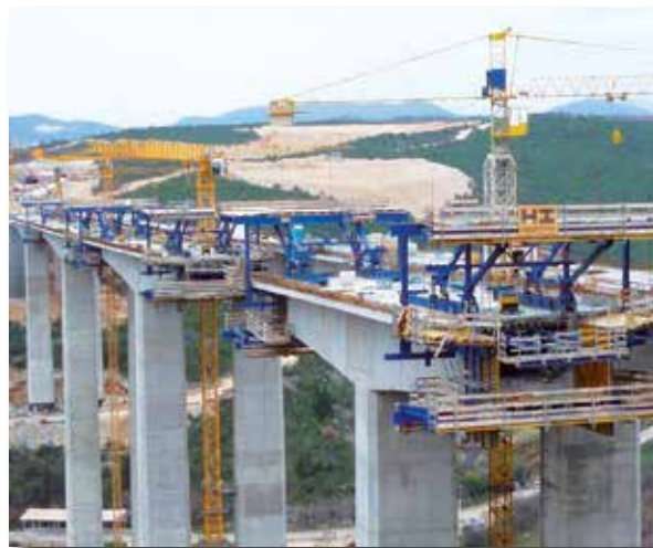
Izgradnja rasponske konstrukcije mosta Studenčica slobodnom konzolnom gradnjom Construction of span structure of Studenčica Bridge by balanced free cantilevering
