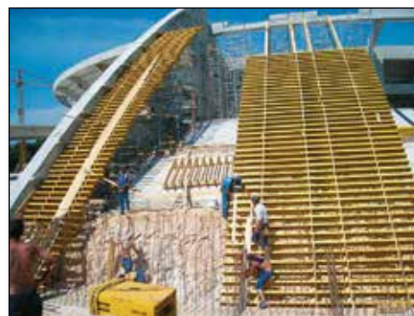
Figure 8. Placing of formwork and scaffold
