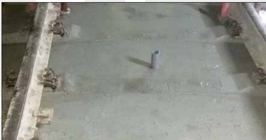
Figure 9. - Placed concrete with treated surface
