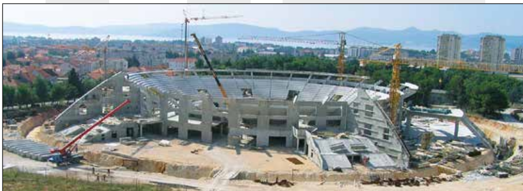
Figure 7. Site view before starting works on dome
