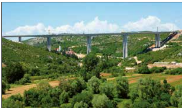
Most Studenčica / Studenčica Bridge
