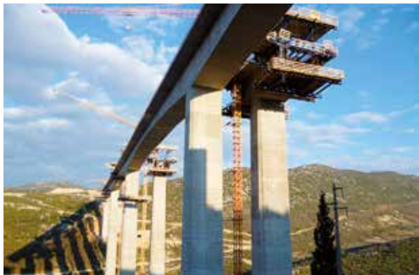
Izgradnja rasponske konstrukcije mosta Studenčica slobodnom konzolnom gradnjom Construction of span structure of Studenčica Bridge by balanced free cantilevering
