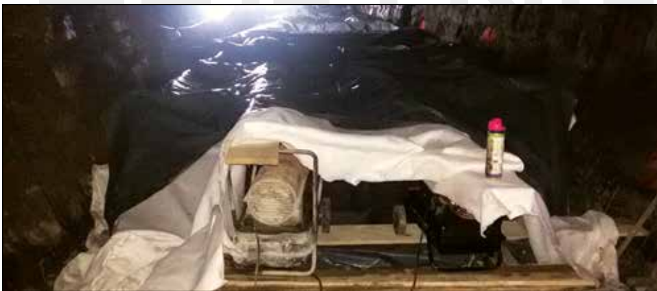
Figure 11. - Curing young concrete by heat using guns
